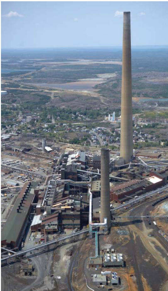
A view over Vale's Coppercliff nickel mine in Sudbury, Canada. The Sudbury area has become a hotbed for mine technology development in recent years. (Photo: Vale Agency)
